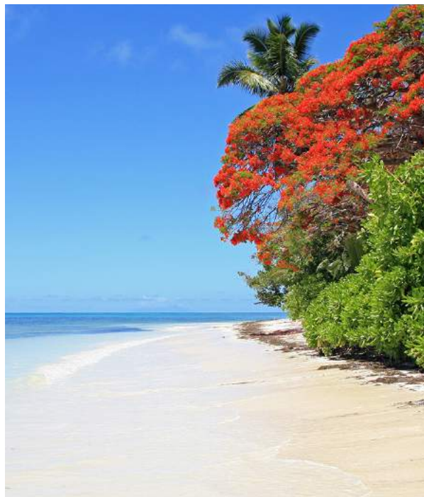
The dike, Source d'Argent cove
